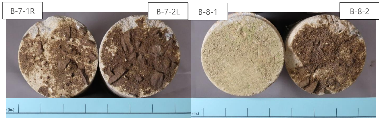
Figure 2. As-received appearance of exterior surfaces of the four core samples. Cores B-7-1R, B-7-2L, and B-8-2 were extracted in the waterline fluctuation zone, whereas Core B-8-1 was extracted at a higher elevation on the bridge pier.
