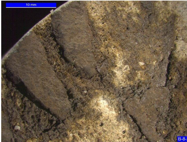
Figure 3. Brown discoloration on the exposed surface of coarse aggregates and paste.
