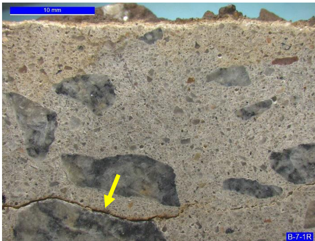
Figure 9. A separation (arrow) near the exterior surface of Core B-7-1R.
